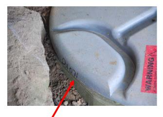
Vent opening is on the underside of the lip.
